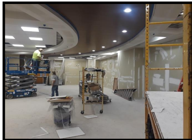
Birmingham VAMC Front Entrance Progress
